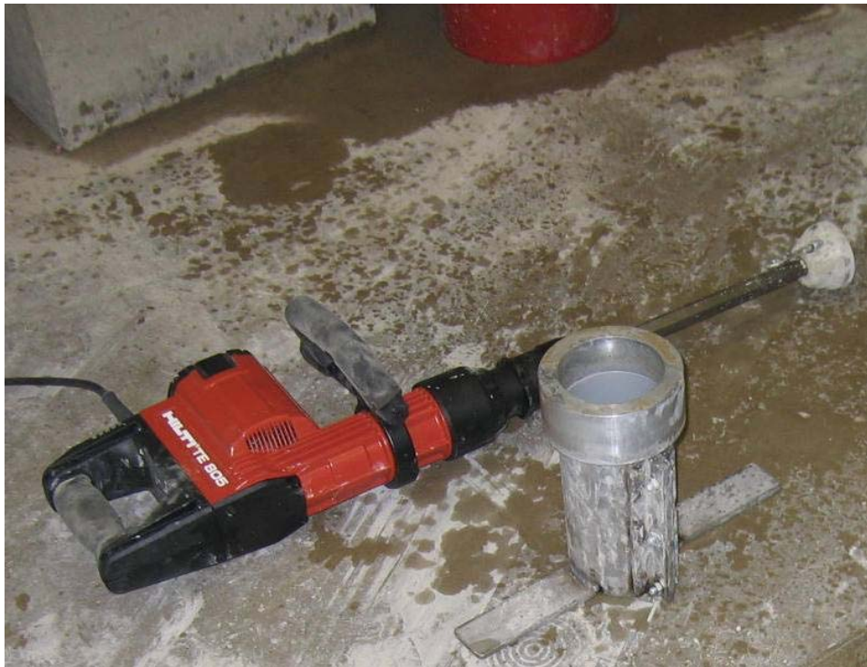
Figure 24 Compacting hammer, steel sleeve and a cylinder
