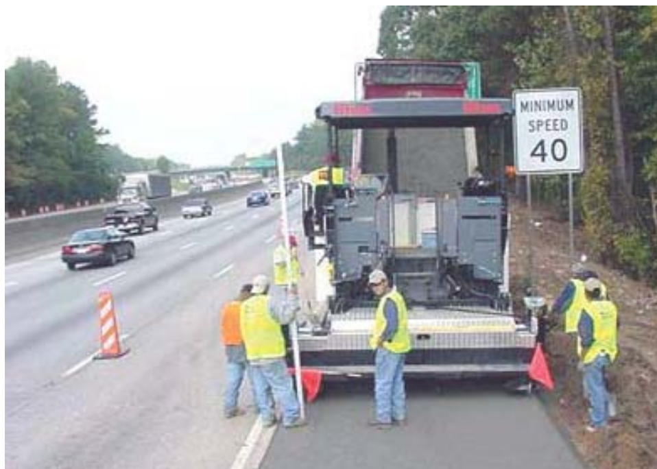
Figure 3 RCC used as Pavement shoulder in Atlanta, GA, USA [5]
